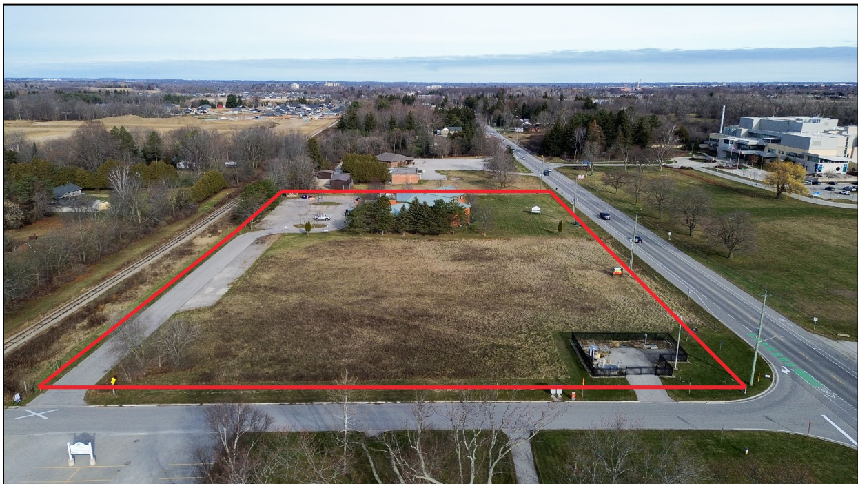
Figure 2 – Subject lands (looking north from Karen Street)
