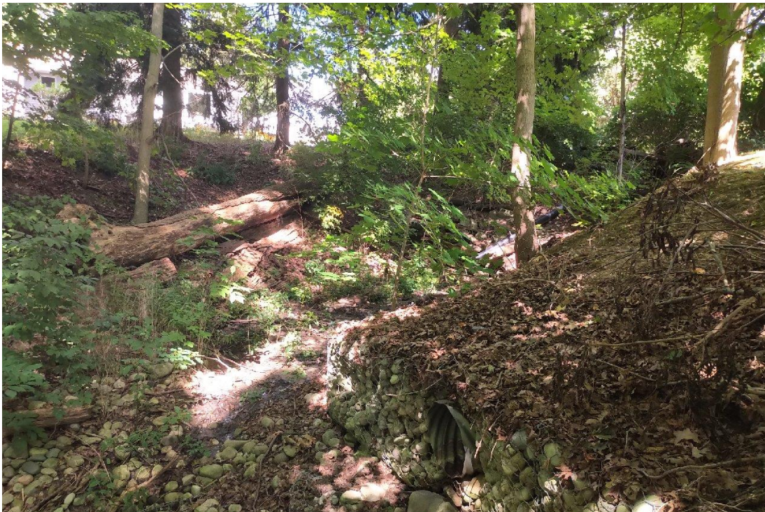
Photograph 4 – Looking north from toe of ravine slope near driveway to property at 279 Hill Street. Note drainage pipe and gabion baskets to the east.
