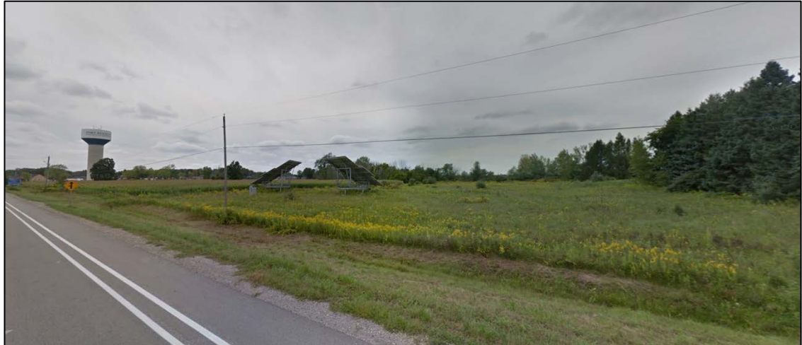
Figure 5 – View on East Road Looking Southwest Towards Vacant Residential Lands owned by Wastell Developments Inc.
