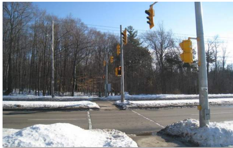
Mid-block Pedestrian Signal – Guelph, ON (Source: MMM Group)
