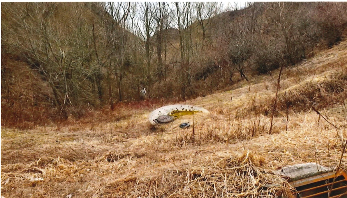
Looking downstream (south) from Barnums Gully Line at first 1997 drop manhole south of road This manhole structure is also the outlet for the Dell Drain Branch G
