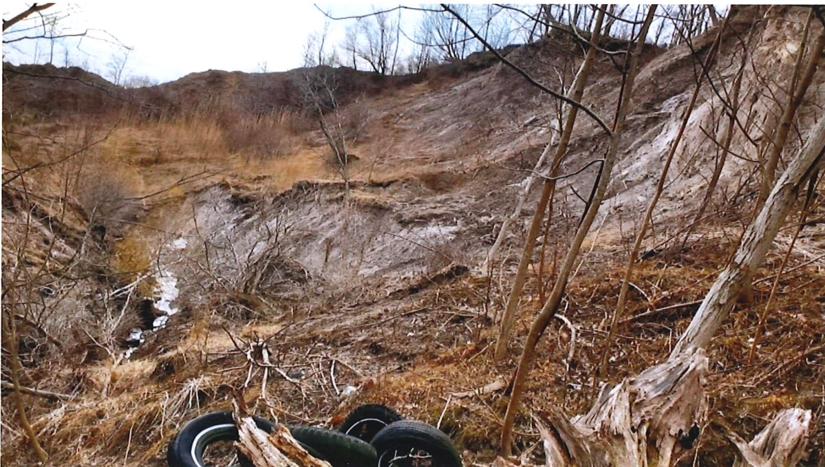
West side of ravine standing on pile of tires at Station 0+100 looking downstream Right side of photo shows upper slope failure area on west side of ravine that is not connected with the flow in the bottom of the ravine on the right side of the photo
