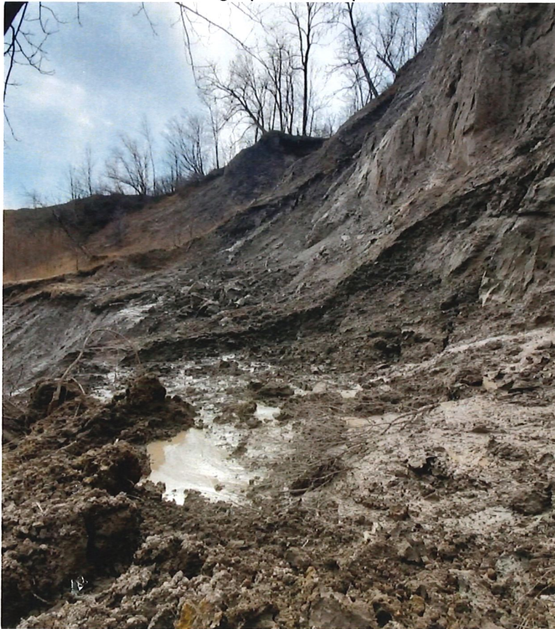
West side of ravine showing top of bank failure due to groundwater seepage in lower part of photo
