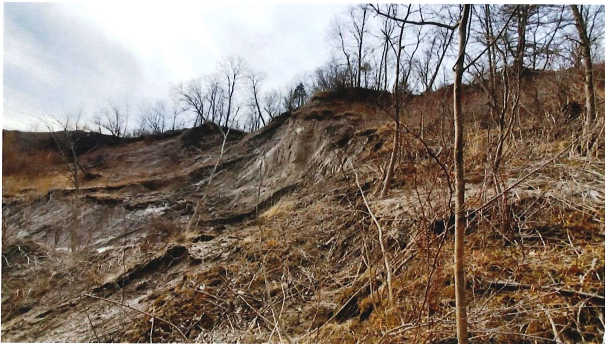
West side of ravine showing upper slope failure area not connected to flow in bottom of ravine
