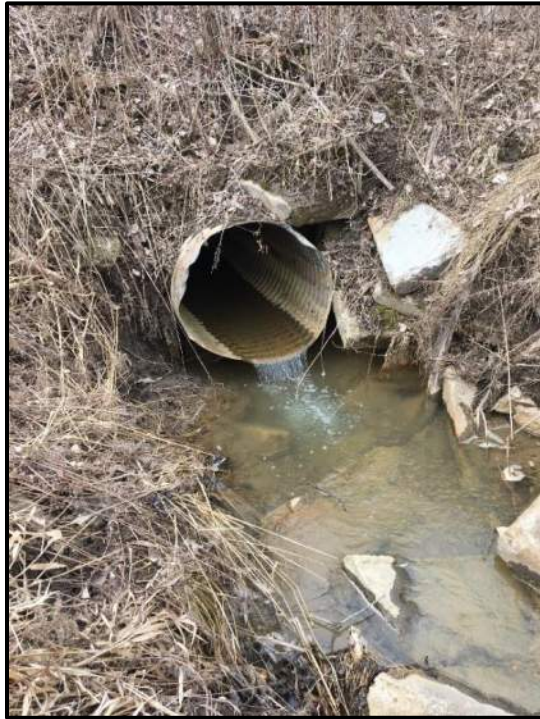
Photo 1: Looking west at the outlet of the CSP culvert within the Lake Road Diversion Drain. Note the perched culvert, restricting potential fish migration. (April 2018).
