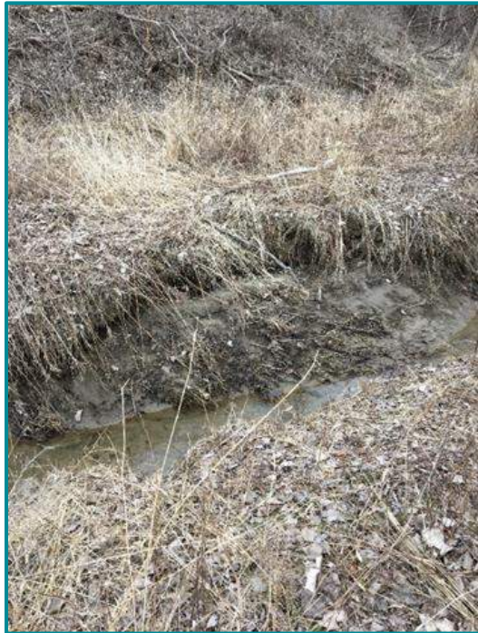
Photo 3: Evidence of bank sloughing in section of Drain before bending east beside golf course. (April 2018).
