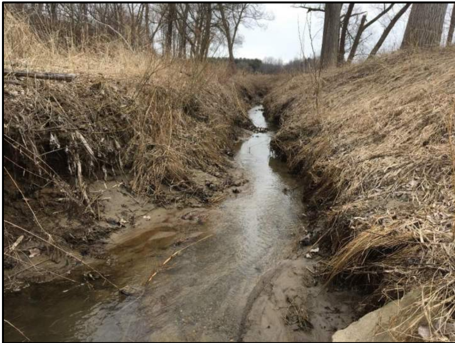
Photo 2: Looking east, Looking east, downstream near the upstream extent of the watercourse. Note the undercut and eroded banks, and shallow, flat watercourse (April 2018).
