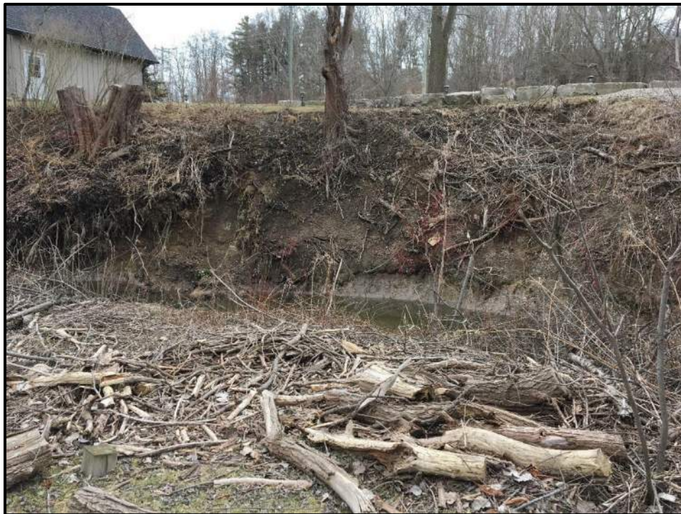
Photo 4: Significant erosion along slope. This section of watercourse is to be realigned. (April 2018).
